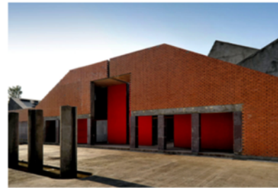
Fig. 1. Brick School, Pune
