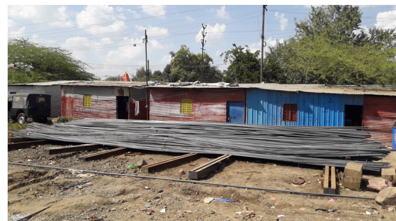
Fig no. 11 Steel reinforcement for construction kept in front of shelters which could harm the children.
