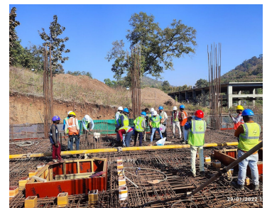
Figure 1: Workers engaged in construction
