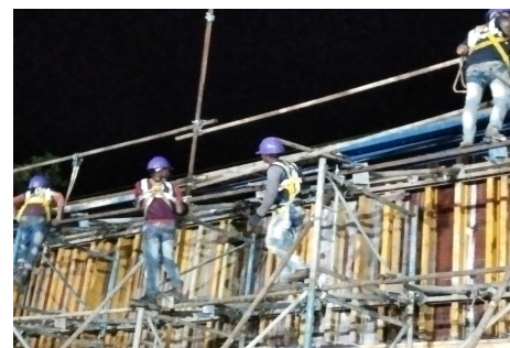
Figure 5: Workers engaged in construction
