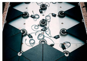
Fig 33 : pavegen details Detail of installation of tiles**
