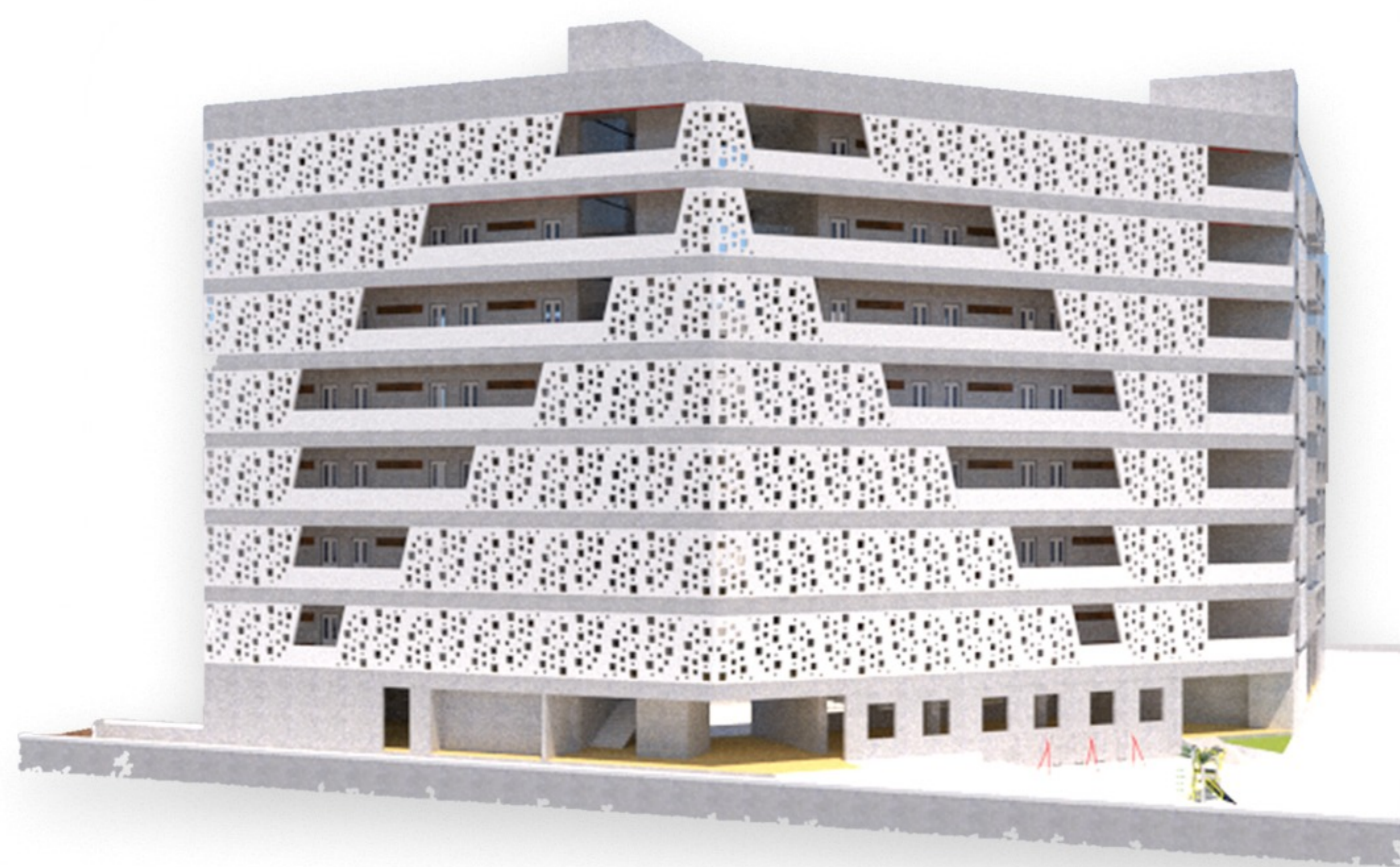
SOUTH AND SOUTH - WEST FACADE
