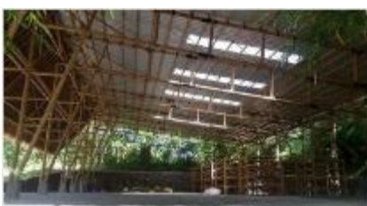
asall ball engineers bamboo structure capable of covering 543m2 every detail of the construction, and particularly its connections, have been carefully designed by a senior
