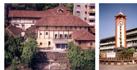
Fig.5 Vernacular construction materials
