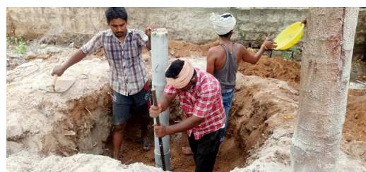
Fig.45. Modular rainwater harvesting system
