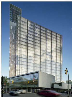
Fig 6.1.5 Manitoba Hydro Place
