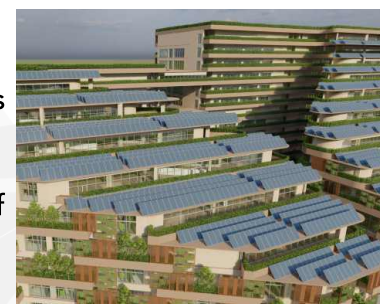
Fig 52 : Rooftop solar panels
