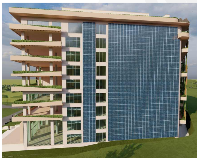
Fig 25 : West wall solar panels
