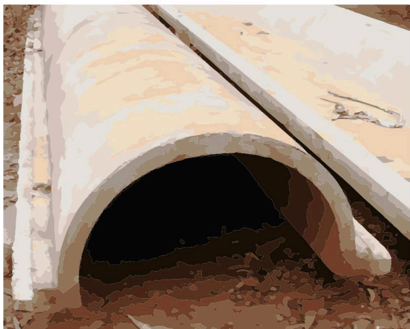
Fig 6.6.5- Ferrocement Vault
